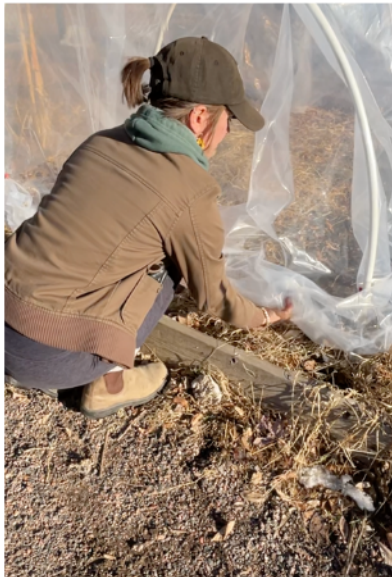
Step 9 - Roll any extra plastic and secure it with bricks or pavers.
