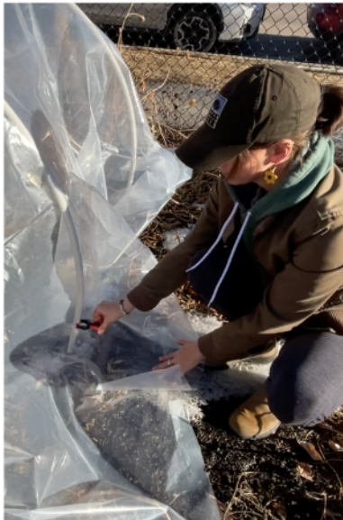
Step 8 - Secure the plastics using your spring clamps at the bottom of all three arches. Be sure to secure both sides of the frames.
