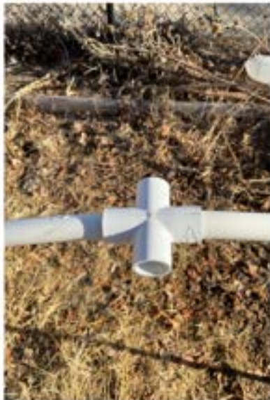
Step 5 - Use the cross fitting Charlotte pipe to connect the two PVC pipes in the middle of the bed to form the middle arch. You should now have 3 arches.
