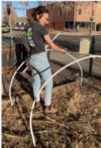
Step 6 - Connect the arches with the 36" PVC pipes and the "T" Charlottes to form a stable structure.
